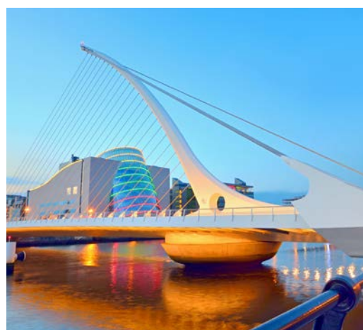
Samuel Beckett Bridge - Dublin Quay
